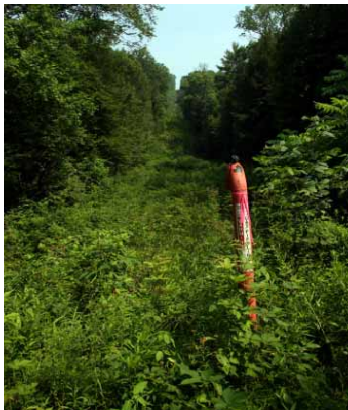
Gas pipeline through SGL 215
