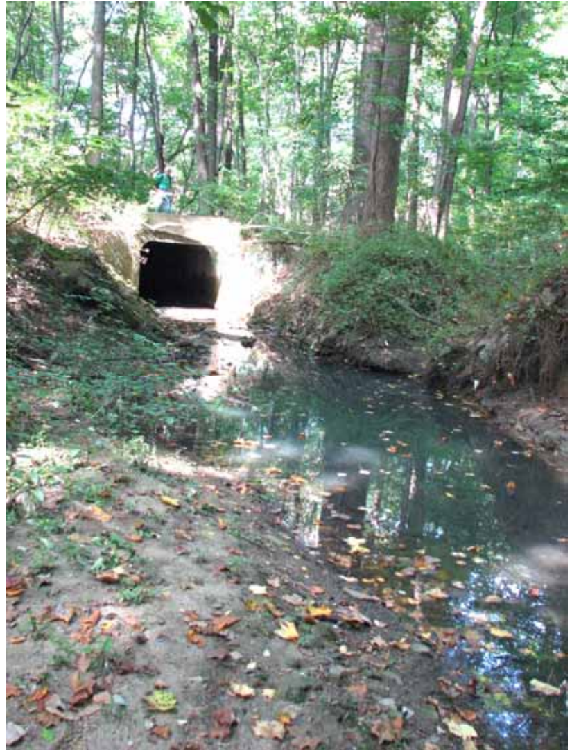
The large stormwater outfall culvert in Bayberry Creek Upland Forest. The adjacent streambanks show the erosion effects of the surge in water levels associated even with small rainstorms.
