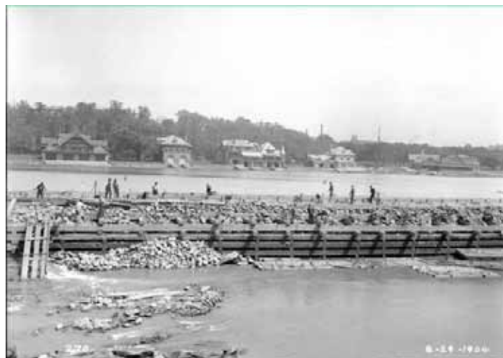
The Fairmount Dam under construction in 1904. This dam, and dozens more along the Schuylkill River and its tributaries, severely impacted the fishery and water quality in Philadelphia.
