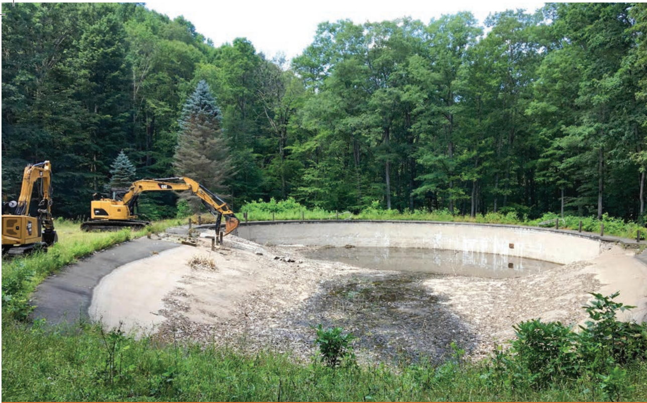
Top photo: pre-construction photo of a large cement swimming pool that was restored to a natural spring-fed pool and wet meadow. Below: shown two years post-construction.
